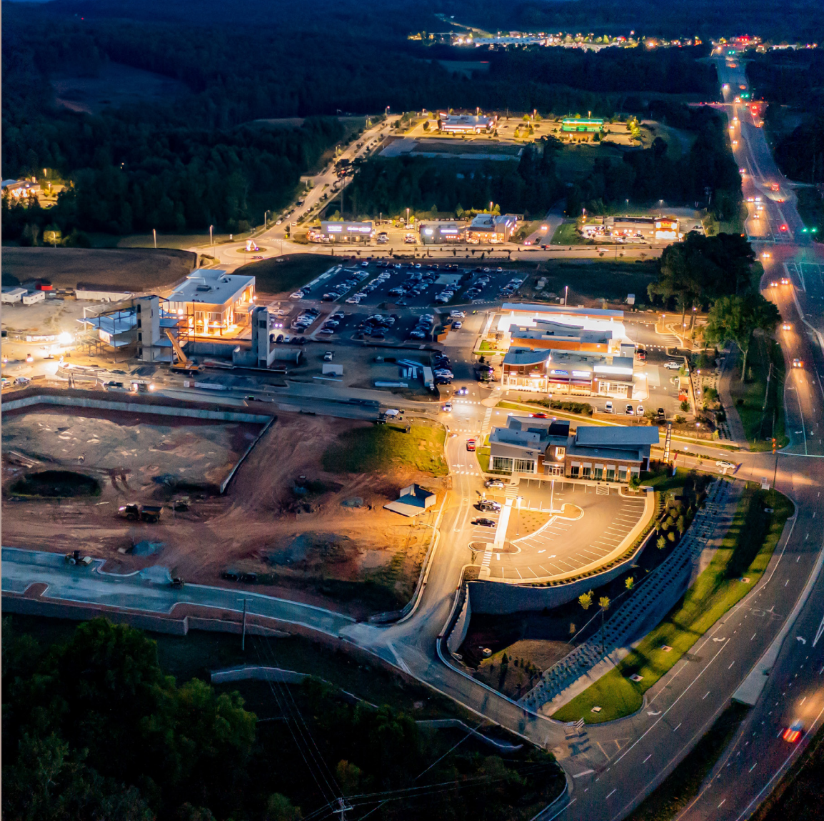
Chatham Park (under construction) at night. Chatham County Public Information Officer
