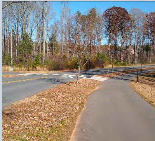
Top: A passenger boards Chatham Transit bus in Pittsboro (source: Chatham News Record) Bottom: A Town of Matthews roadway example with a shared use path Right: Example of NCDOT cross-section (typical section No. 3D) with a shared use path
