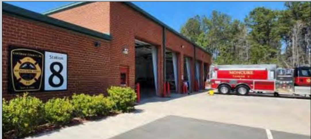
Top Photos: Moncure school and gymnasium. Bottom: Moncure Fire Station.
