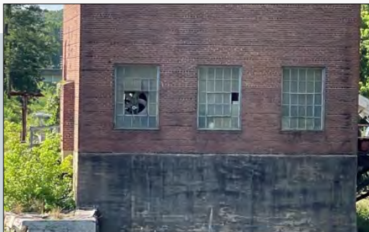
The Lockville Dam, Canal, and Powerhouse at Old US-1 and the Deep River are listed on the National Register of Historic Places.
