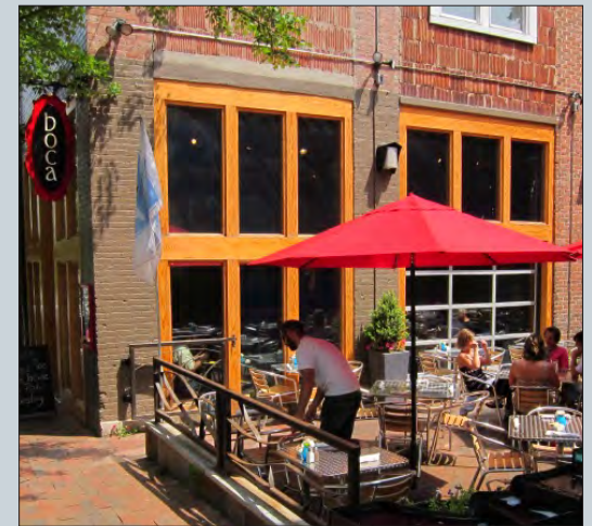
Top: Recent work has occurred to restore and repurpose old commercial buildings in historic Moncure. Bottom: Thoughtfully designed infill development can bring new retail and dining opportunities to the local community.
